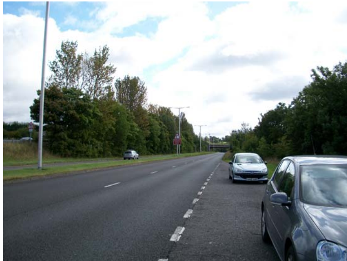
Plate 4 – A4023 Coventry Highway adjacent to Development Site
