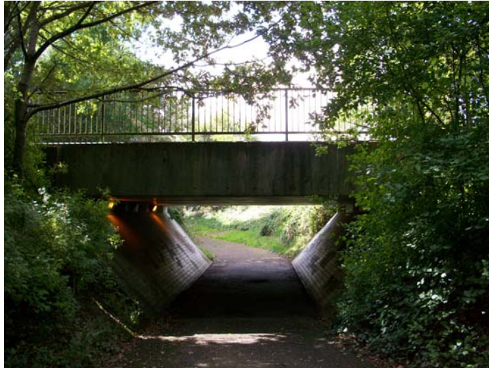
Plate 9 – Typical underpass under Far Moor Lane
